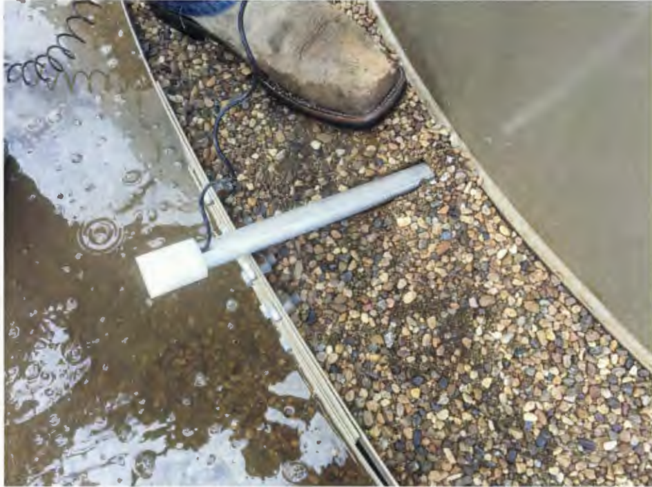
Anode partially installed under tank
