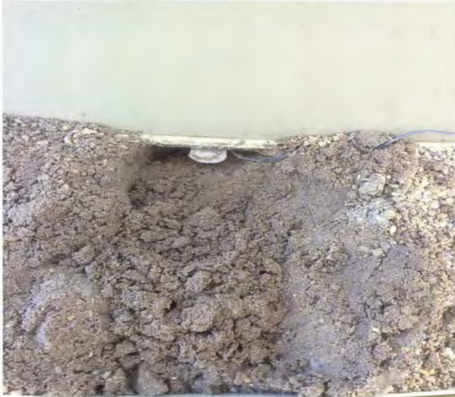
Anode fully installed under tank
