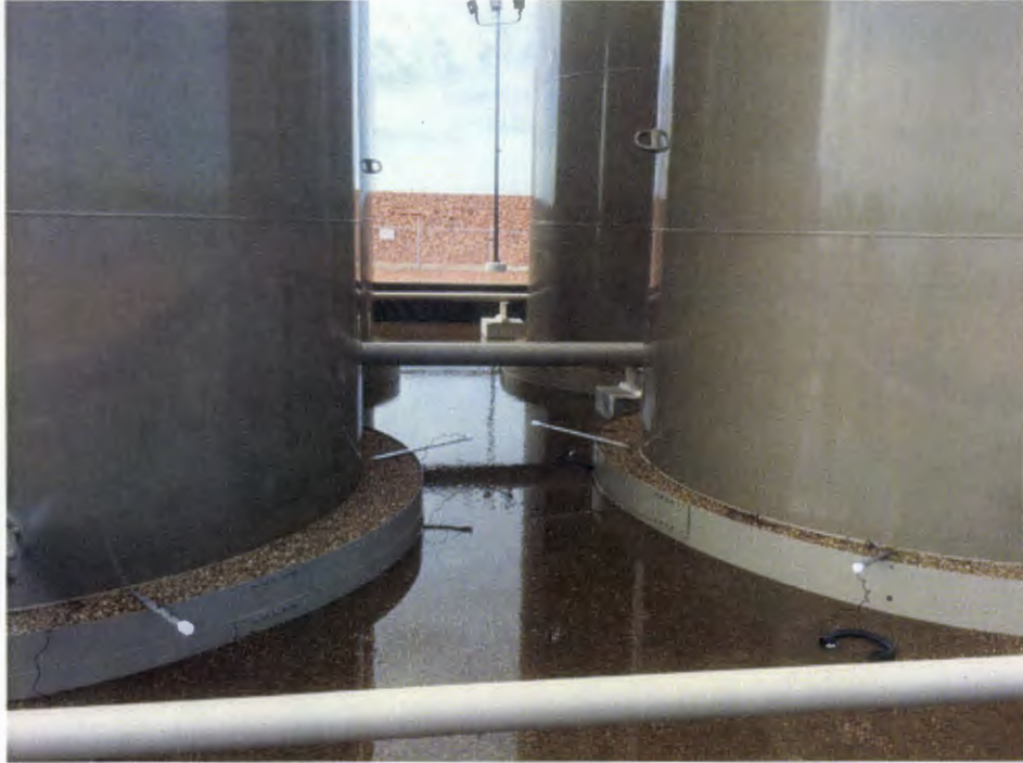
Anodes as laid out under the tanks
