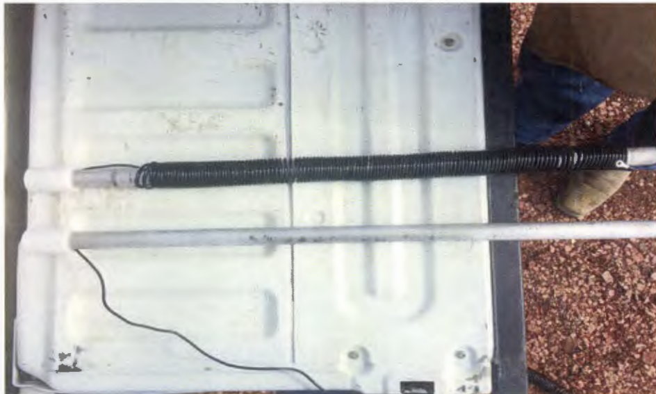
Anodes Prior To Installation
